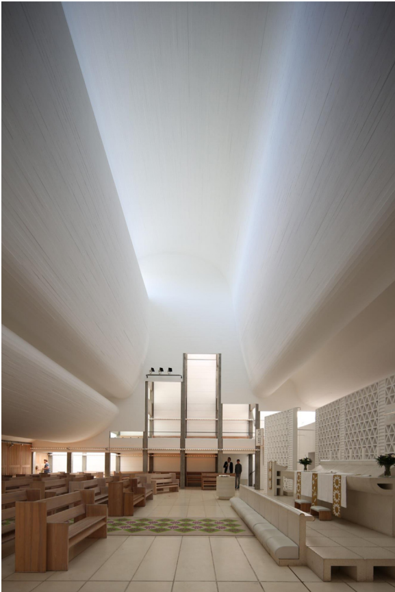
Fig. 17 Photograph showing the completed shell by the situ spray concrete and prefabricated angular units for walls and floors at main church of Utzon's Bagsværd Church. From authors' own photograph.
