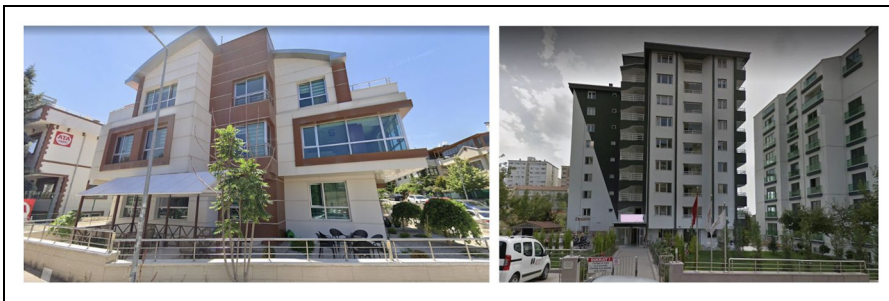
Figure 1. Overview of the nursing homes, highlighting differences in building size.
