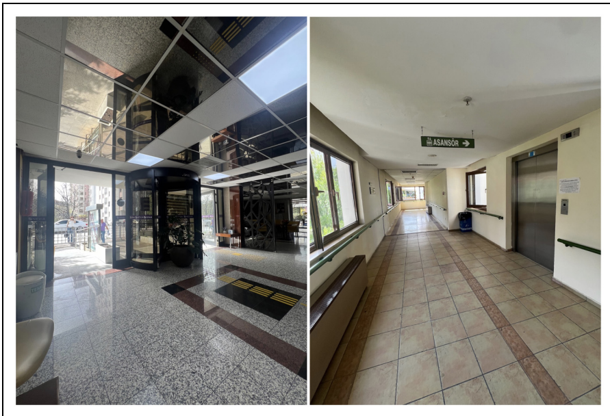
Figure 7. Prosthetic aids: Wide hallways with handrails and automatic doors.
